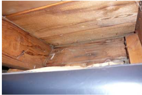
Over cut trim water damage potential
