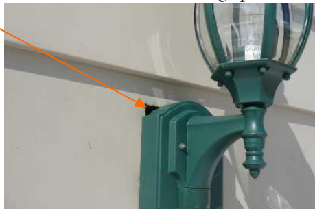
Over cut trim water damage potential
