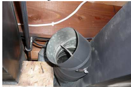
Missing heat duct cover
